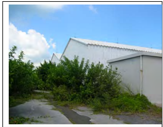
T&C building. Southern facade (2006)
