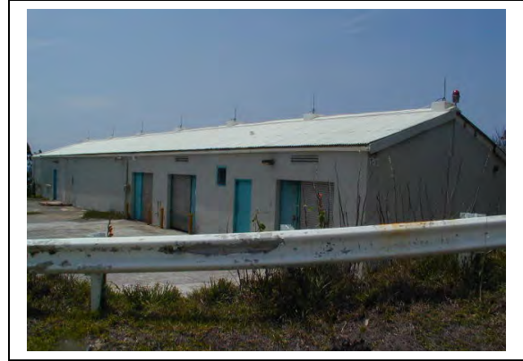
Workshop shortly after station closure. Southern facade (2006)
