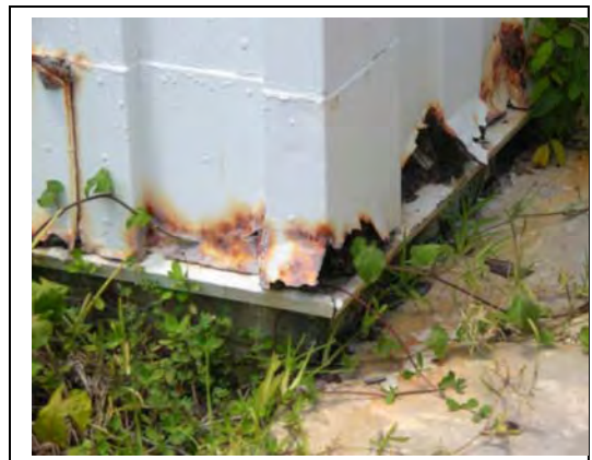
Corrosion of prefabricated cladding on all section of the building (2006)
