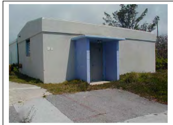
Pumping station just after closure (2002)
