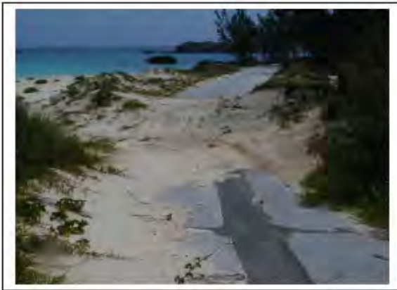
3. View along access road showing storm surge over main access road.
