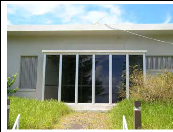
Operation Centre front door (2006)
