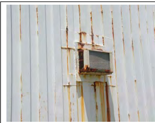
Corrosion of prefabricated cladding on all section of the building (2006)
