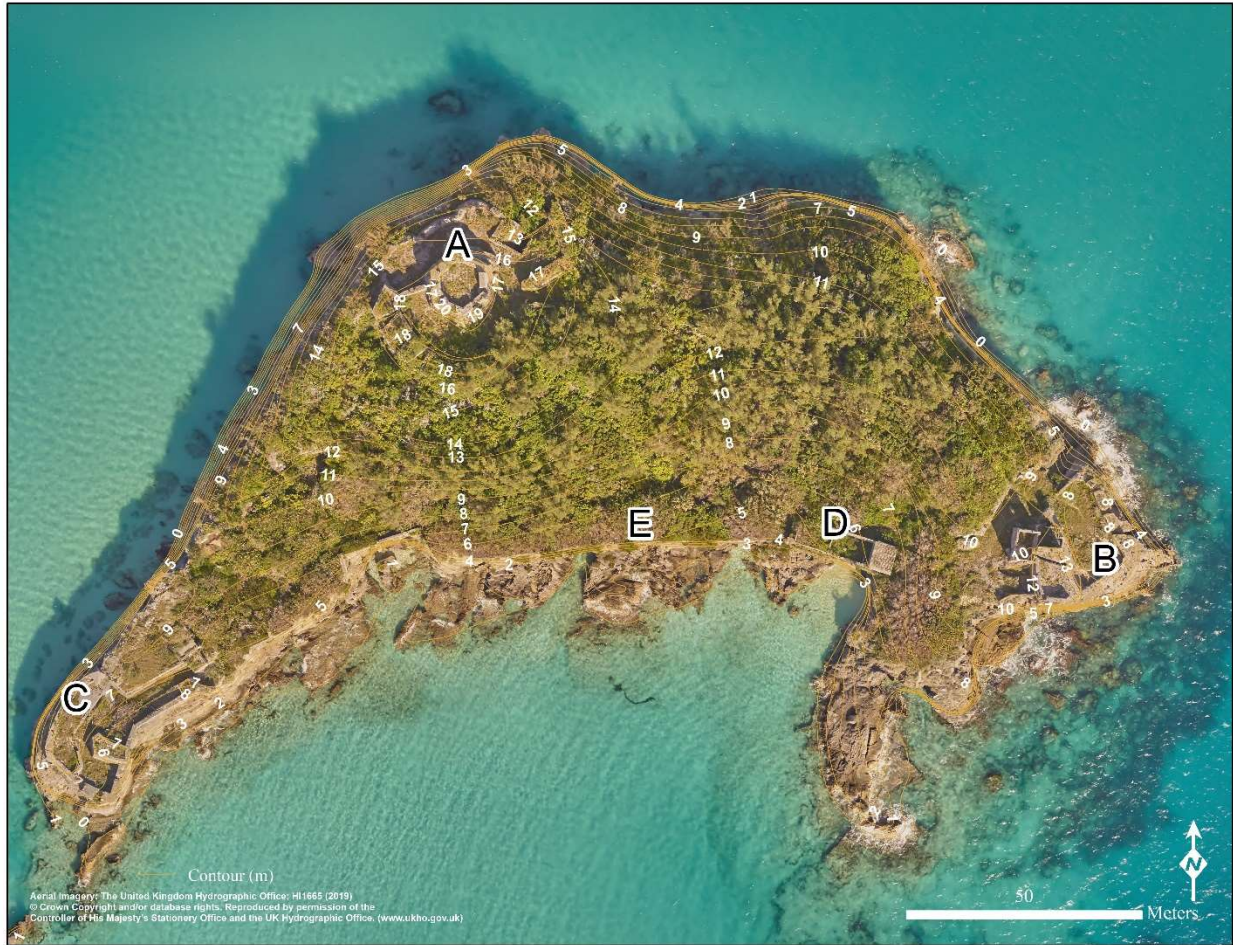
Figure 3. Aerial view of Castle Island showing fortifications and elevation contours. A. Devonshire Redoubt, B. Seaward Fort, C. Landward Fort, D. Barracks Building, E. Curtain Wall
