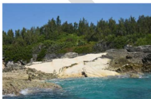
1 Sloughing of coastal surface to small peninsula south of King's castle.
