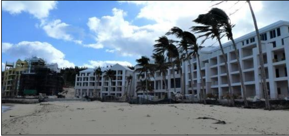
The St. Regis hotel under construction (Photo: Alison Copeland)
