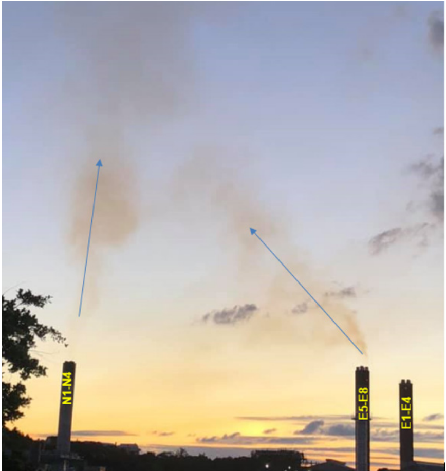
Figure 2. Photograph of the exhaust plumes from the four new NPS (N1-N4) engines compared to one engine operating from the EPS (E5-E8). One theory is that the exhaust from fewer engines may not get as lofted vertically (i.e. EPS) compared to when all four engines are operating in a stack (i.e. NPS) thereby leading to an apparent topographical downdrafting effect over Langton Hill.
