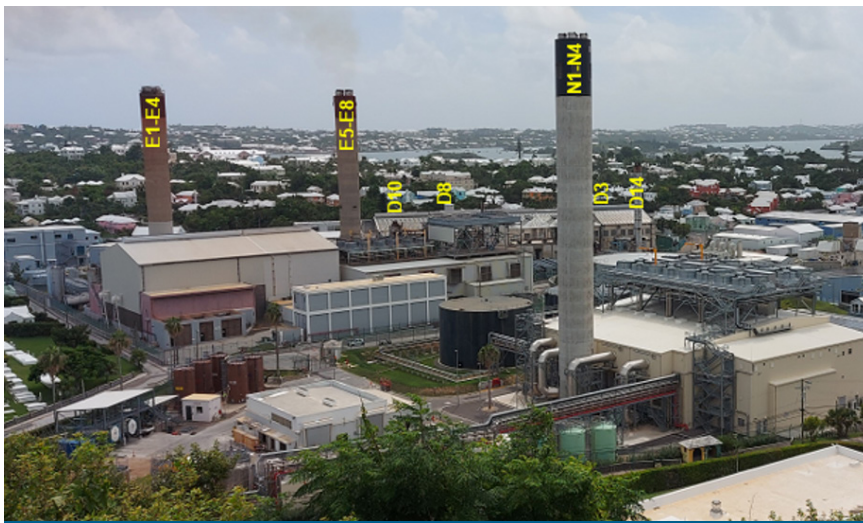
Figure 1. Aerial view of the BELCO power plant from Mount Hill showing all base load engine stacks.
